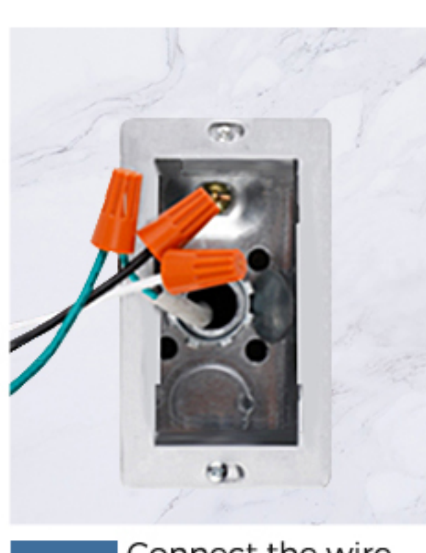
STEP2 Connect the wire with the connector
