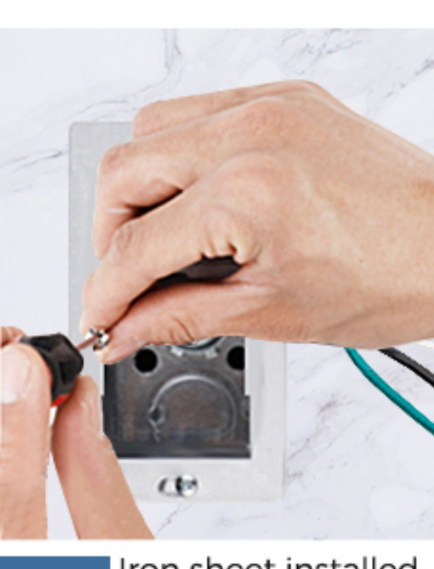
STEP1 Iron sheet installed in the junction box
